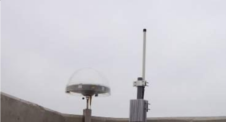
GNSS & Comm Ant installation
