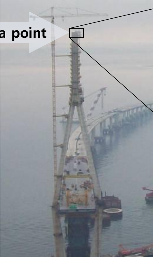
Main Bridge Tower
